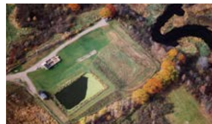
Figure 2 – Aerial view of lagoon converted to SBR and sludge holding pond.
