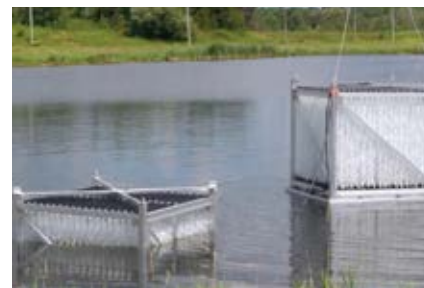
Figure 1 – Biocord reactor installation.
